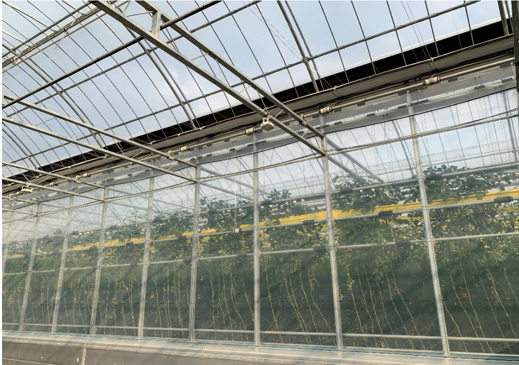
Picture 3. Mid-Tech Plastic Greenhouse for Tomatoes with an Automatic Roof Vent
