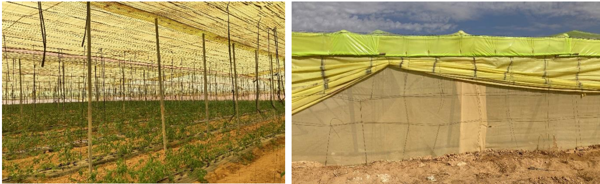
Fig. 28 & 29 Screening and side ventilation in Canarian greenhouses in Biskra
