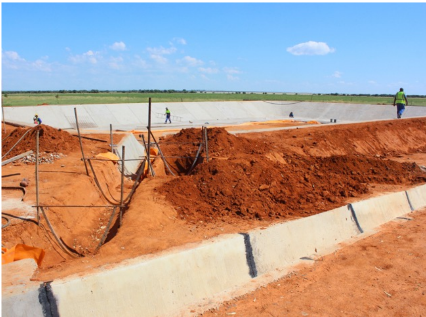
Construction of a basin for emerging farmer
