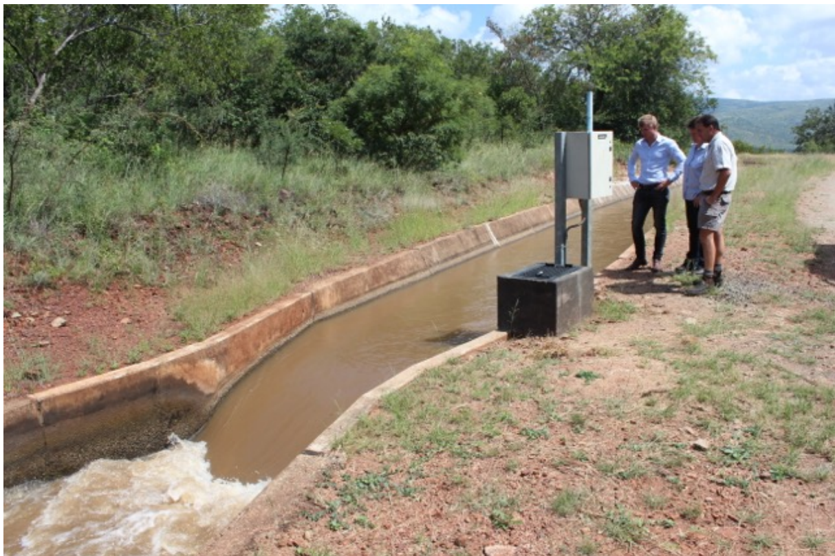
Irrigation canal, erosion of lining (left hand side)
