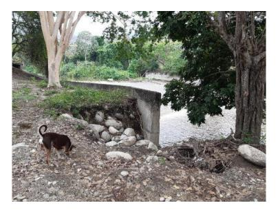
Figure 4-6 Damage to the river bank of Río Sevilla just south of the main intake of ASOSEVILLA, damage caused by the 2021 flood. (picture of Acacia Water, April 2022).
